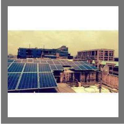
Solar Power Plants
